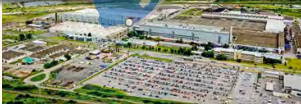
View of the plant: Around 4,000 employees work in Uitenhage.
