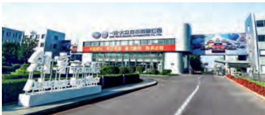
Gateway to the plant: a look at the plant premises in Changchun.
