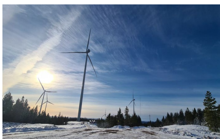
New wind farm in Skellefteå, northern Sweden: Volkswagen supports electricity generation for 27,000 households
